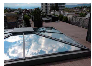
Dachfenster in Zürich
